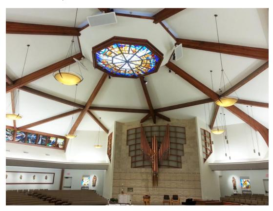
The ceiling has a gentle slope, finishing at the apex in the middle of the room, with a stained glass feature, located at the bottom of a large, octagon soffit. The eight major facets of the ceiling form a giant parabolic reflector that focuses sound on the floor, near the center of the room, where the Altar table is located.
