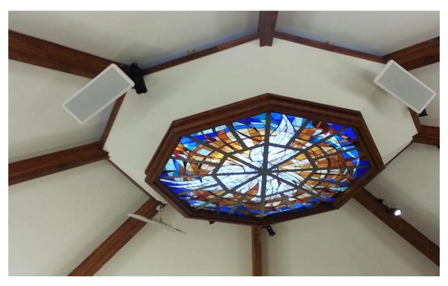
Given this spacing and aiming, we had significant horizontal overlap between the perpendicular pairs of panels. This overlap produced an audible "thickening" of the sound in the low-mid range frequencies around 200 - 400 Hz, but there is no noticeable, mid-high comb filtering issues in the overlap zones.
